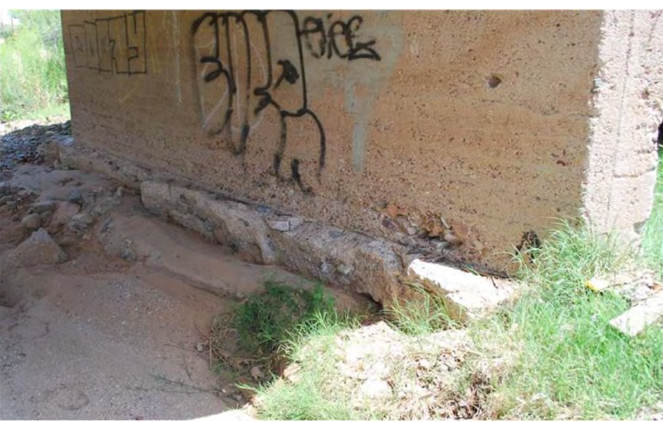
EXISTING PIER FOOTING/CAP
