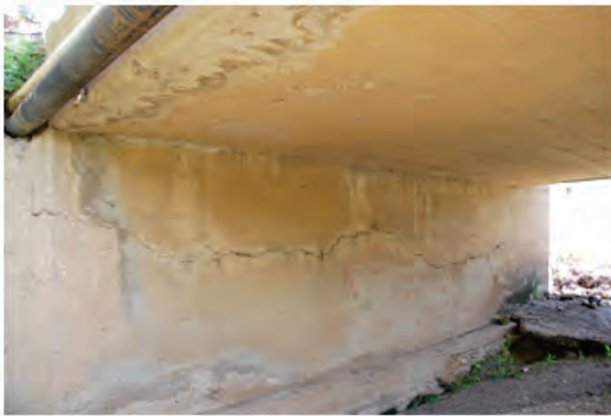
Typical pier vertical cracks
