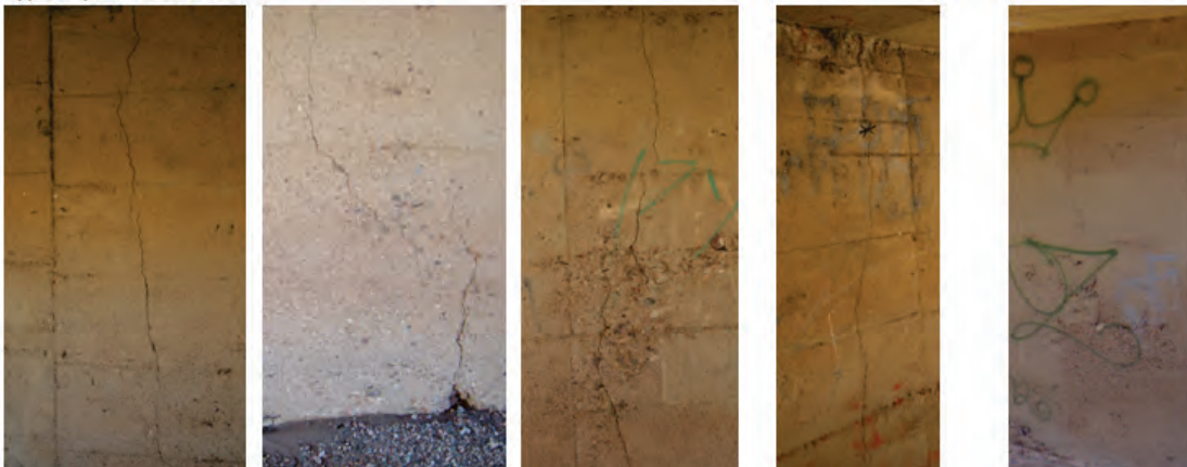
Typical pier vertical cracks
