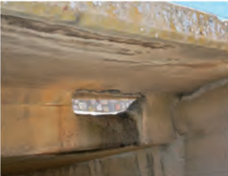
Delaminating Drainage Retrofit, North end, east face
